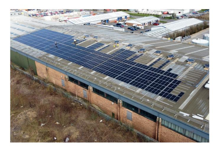
efficiently and, most importantly, delivering in line with the customers objectives. Since the plant went operational, Faerch have recorded annual CO, savings of over 450 tonnes per annum directly attributed to the solar energy generation. Average annual savings on electricity are in the range of £85,000 or £2m+ over the lifetime of the system.
