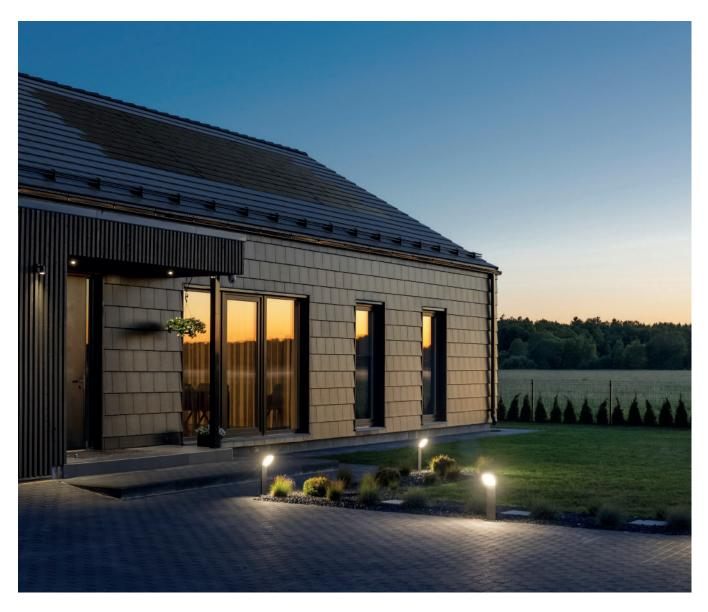
frame. Panel production is left to those who do it best, Tier 1 manufacturers. Adding the frame does not void the original warranty but does make the panel sturdier. Tackling  $installation\ complexity,\ Solar stone\ solar$ roofs are mounted directly on the wooden battens without any expensive mounting systems. Standard 80m² rooftop can be easily fitted with panels in just one day.
