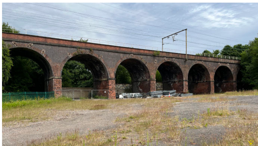
The initial site visit
