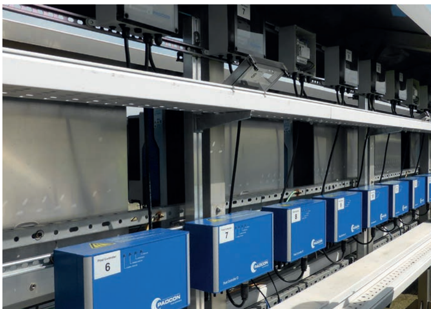
Installation example: Installed Float Controller CI for the regeneration of degraded PV modules.
