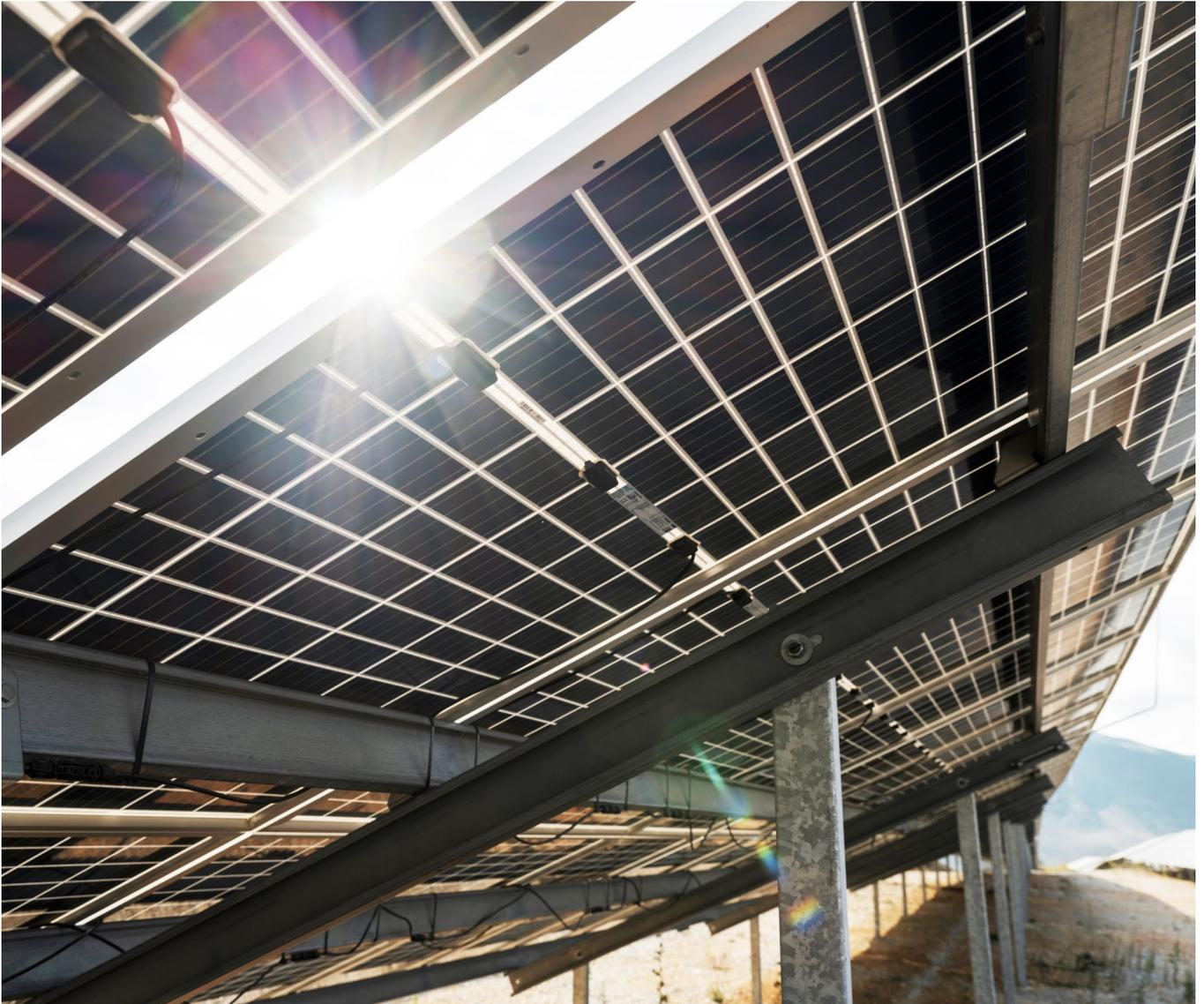
In a 200 MW large-scale PV plant there are more than 1 million connectors that could potentially fail if not assembled and installed correctly
