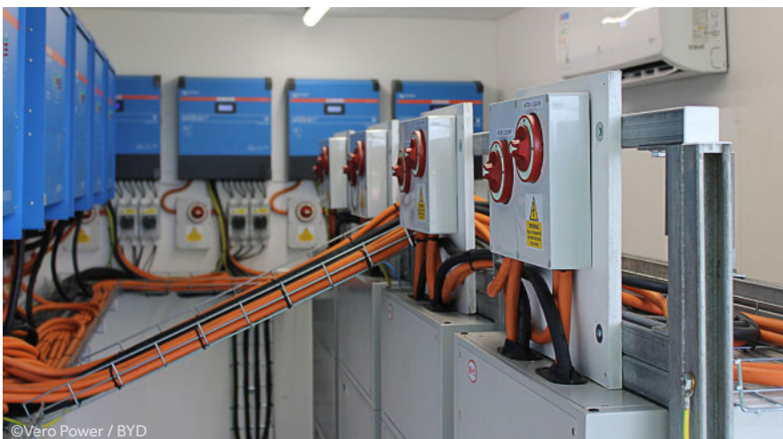
Energy management equipment and eight 15 kWh BYD Battery-Box LVL battery storage systems
