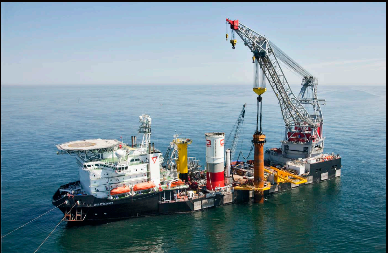
The first ever Mono Piles driven with a vibro hammer in offshore wind
