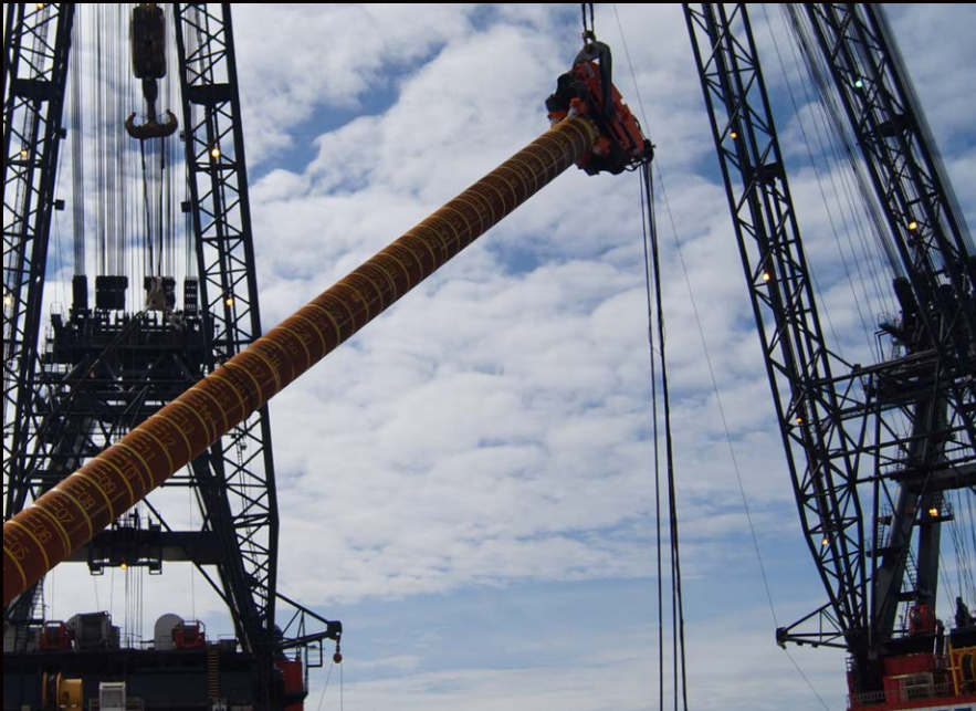
Dual crane upending of a 250t pile
