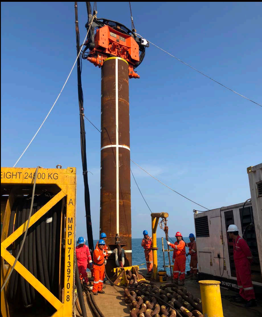
CV-80 VLT-U being used for anchor piles for an FPSO
