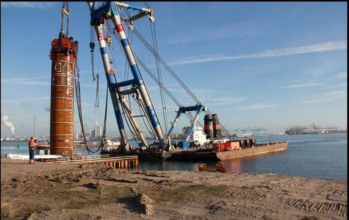
6.5m monopile at the Maasvlakte; 24-meter penetration in 15 minutes net driving time
