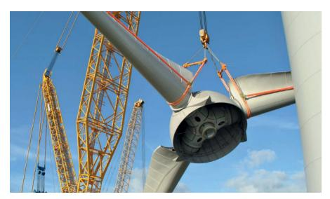
blades to be assembled. The traverse can thus safely take on and handle diverse blade shapes with a blade weight of up to 30 tons.
