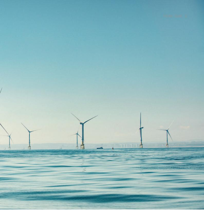
Traditional installation of fixed-foundation offshore wind projects requires foundations that are installed on site, with tower segments lifted into place at the array location, and the nacelle, hub and blades attached thereafter. Major component replacement, if required, would likewise take place on site.
